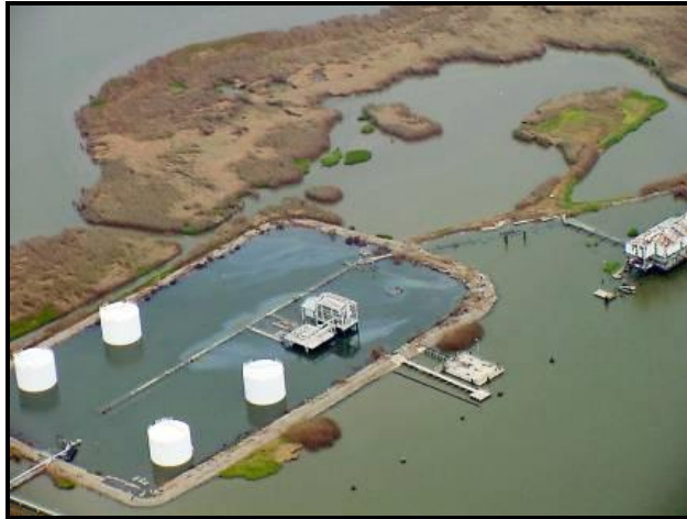
Inundation & corrosion of infrastructure
